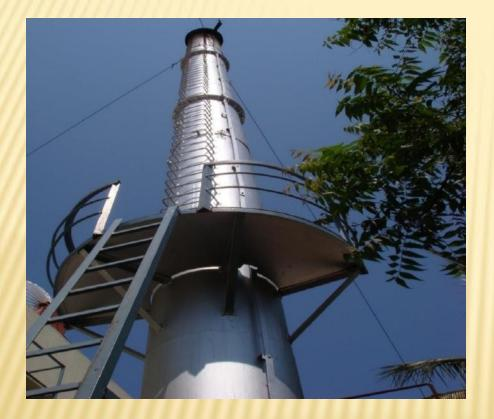
We manufacture the chimney. It is a structure that provide ventilation for hot flue gases or smoke from a boiler
