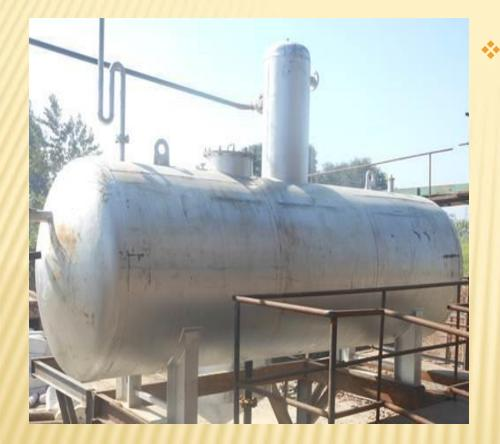
The Deaerator tank acts as a Feed Water Tank to store cold and hot fluid in order to remove dissolved air or non-condensable gases from the fluid.
