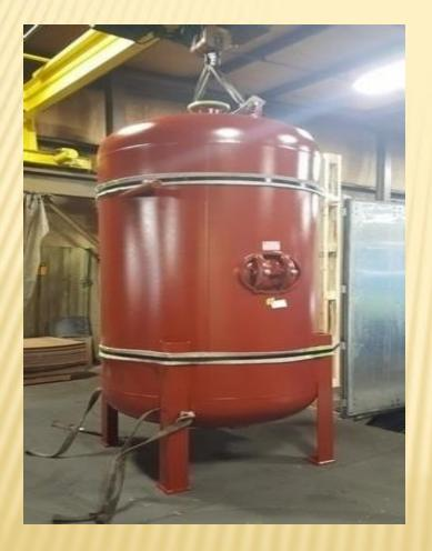
Blowdown tanks for boilers are used as an alternative system for cooling the bottom boiler blowdown. These large tanks retain the blowdown water volume from one blow after the flash steam has been vented to the atmosphere and allow the water to cool down by natural convection over 6-12 hour period. The cooled water will be below 140° Fahrenheit when it is displaced by the next blowdown and forced out of the overflow drainpipe.
